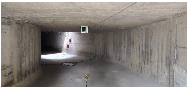
Figure 7 Setup for measuring the available power of a solar cell in an combined sewer overflow outlet pipe (viewed from watercourse exit)
