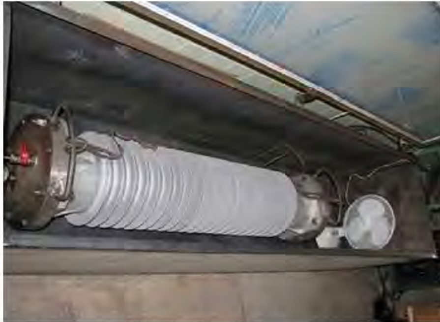
Figure 3 – Isolator testing, Novosibirsk 2008
