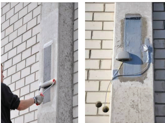
Figure 4: Handling at building site
