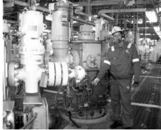
Fig. 1b. Installation of a wireless pressure transmitter in the Grane platform.
