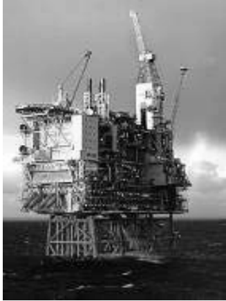
Fig. 1a. Grane offshore platform, operated by StatoilHydro in the Norwegian Sea off the coast of Bergen, Norway.
