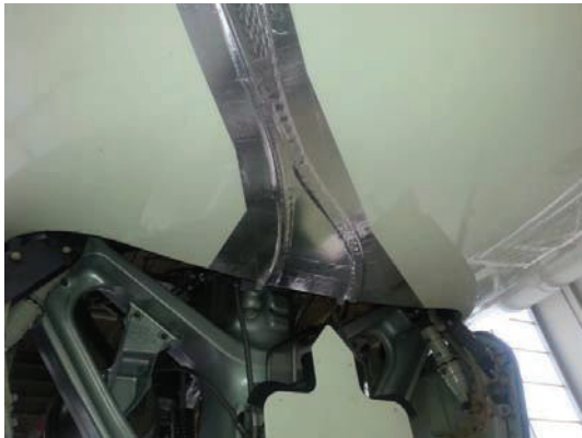
Figure 13. Cable connection to NLG bay.
