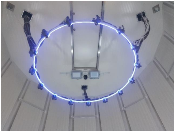
Fig. 4: Spray system in the cooling chamber [3] © DLR
