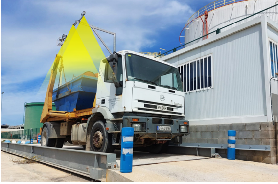
Figure 1: Installation of Clever Sense system at the Port of Barcelona, illustrating sensor placement for optimized waste volume monitoring in compliance with MARPOL V standards.
