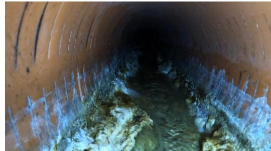
Figure 4: Medium to strong scaling at the bottom, formation of algae
